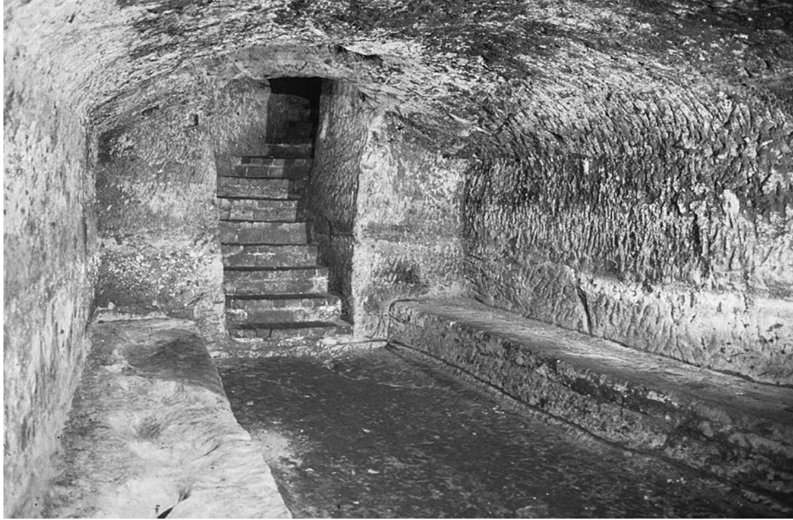
Figure 2 An old beer cellar cave beneath a public house; it is a typical cave with its stairway entrance from the building above. The barrel thralls have been mistaken for beds in some interpretations of the cave's origin.
